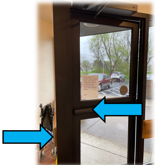
North West Exterior Door
